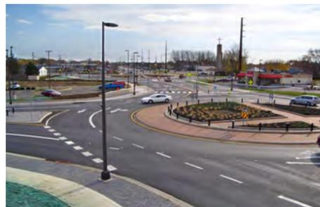
intersections. Burgess & Niple (B&N) designed two roundabouts and one signalized intersection to replace them – an innovative solution that keeps traffic moving through this growing suburban community. The design also minimized right-of-way impact on the surrounding area which includes five schools and numerous businesses.
