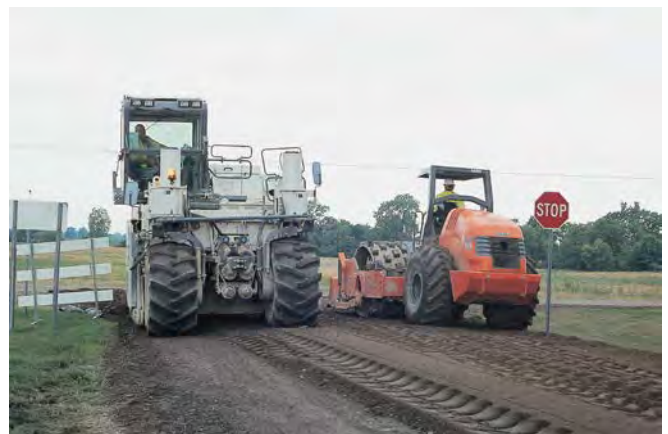
WR 2500 S and Hamm 3412P mix, compact Marysville, Ohio road.
